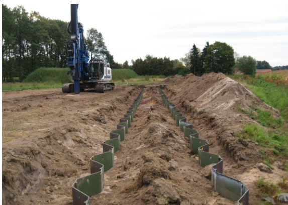
BW 8: Spundwand Widerlager
